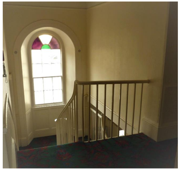
A typical Regency arched sash stair-light window with coloured glass over and frame with motifs
