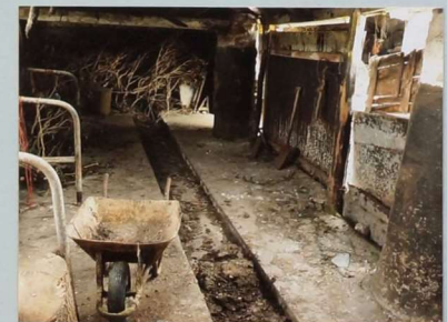
The now deserted cowshed is a conversion of the original open fronted cattle shed. Note the heavy pillars supporting the roof, a feature in several of the local farms.
