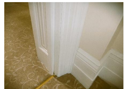
Door frame architrave & high skirting board
