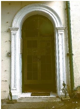
North facing entrance with Regency arch
