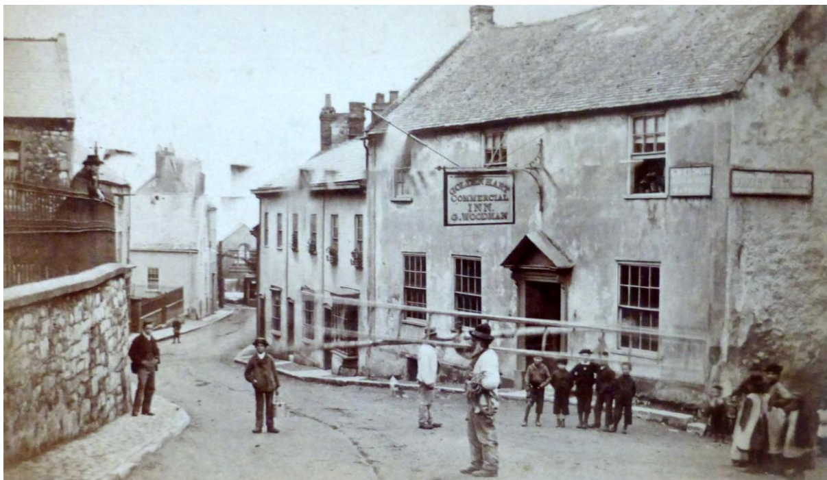
Looking down the southern end of Church Street (Butter Market) in late 1800s
